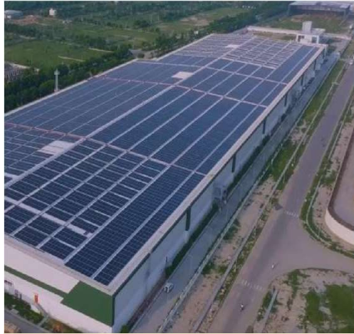
Successfully commissioned solar rooftop plant in Jaipur, Rajasthan.
